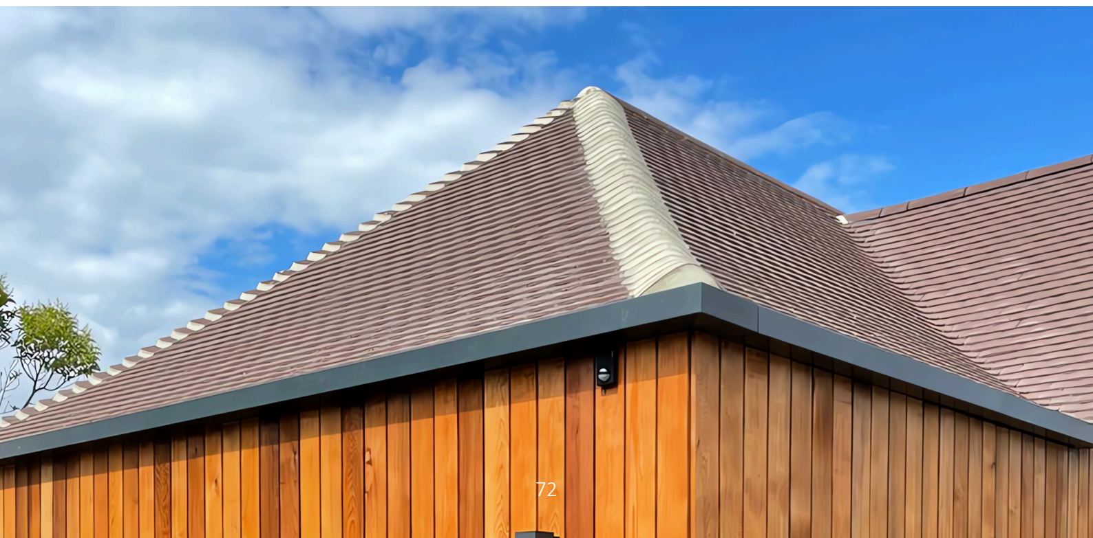
BGC1 — 90° external corner of box gutter
